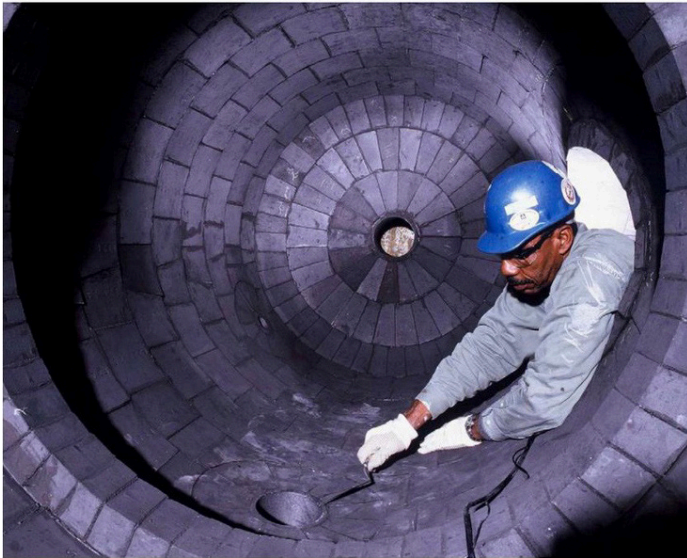
Figure 2. A carbon brick-lined vessel used in phosphoric acid vessels.
