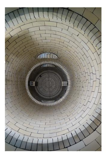
NOTE: All acid-proof brick manufactured conforms to ASTM Spec. C-279.
