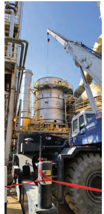
The drying tower bottom and mid section lifted into place.
