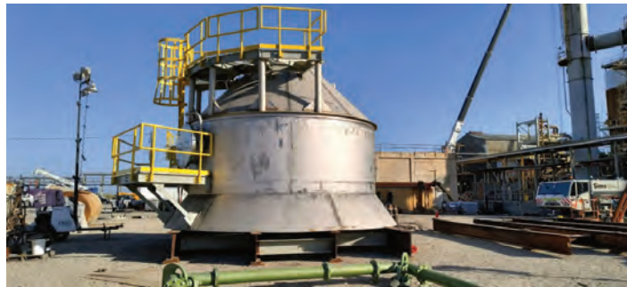
For maximum efficiency, the top section of the drying tower was welded after the internals were installed.
