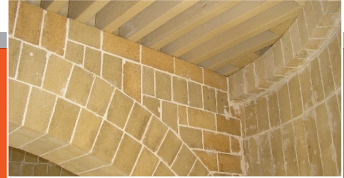
The view from under bar support of tower construction.
