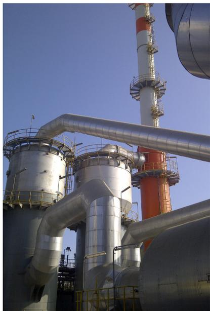
KMT explained to the OEM engineers the idea of injecting resin into the interstice between the brick and the steel shell of the intermediate absorption tower that had suffered the damage. At the time, they were not convinced that an injection of resin could be the solution. They were concerned about the level of acid resistance of the resin in that harsh an environment and the uncertainty of how the interaction of the
